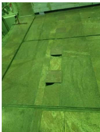
Figure 20. Broken floor area in the Machine Hall of Toktogul HPP (Status in May 2023)
