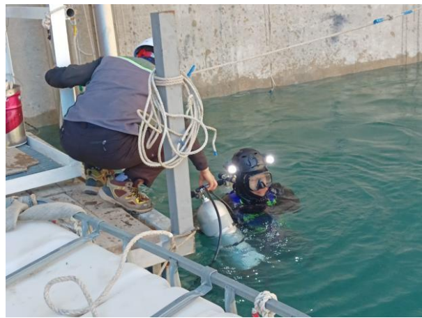
Figure 49. Diving work – installation of aeration pipes of a deep spillway under water (Status in April 2023)
