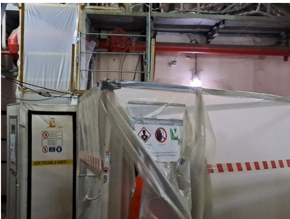
Figure 43. Asbestos cleaning the ventilation system cable gallery (Status in April 2023)
