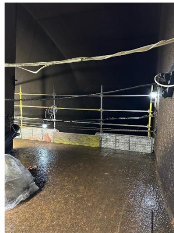
Figure 51. A safety barrier was installed for the construction of scaffolding in the conduit of Unit 3 (Status in May 2023)
