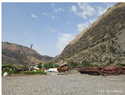
Figure 22. Storage area of dismantled equipment of Toktogul HPP (Status in June 2023)
