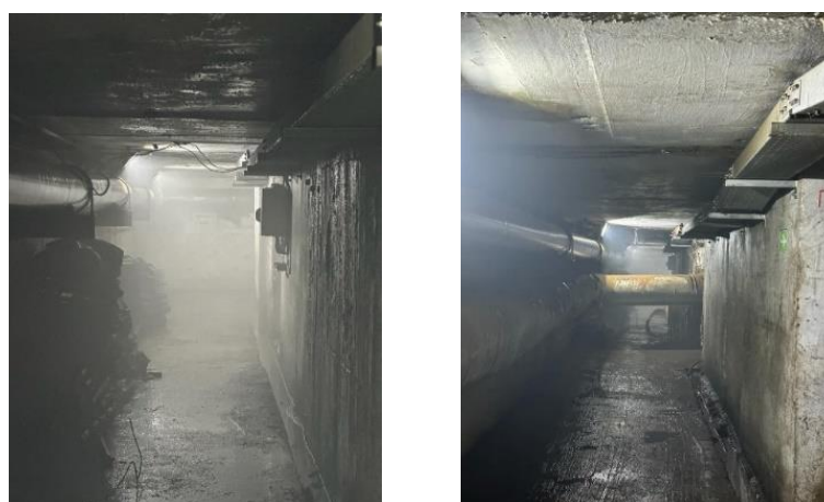
Figure 25. Polluted air on elevation 707 m during sandblasting works of CC ZMEC (Status in June 2023)
