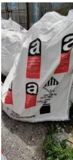
Figure 18. Openly stores asbestos waste bags at Toktogul HPP storage area (Status in 16 May 2023).
