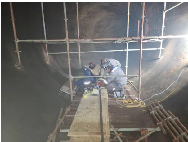
Figure 50. Preparatory work for sandblasting in the Unit 3 conduit (Status in April 2023)
