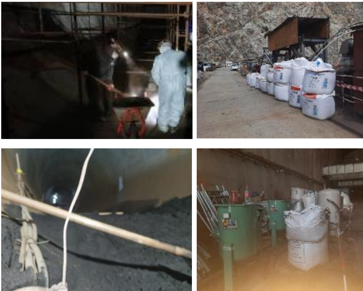
Figure 47. Sandblasting treatment of penstock of Unit 3. Transportation of abrasive debris to the landfill. (Status in May-June 2023).
