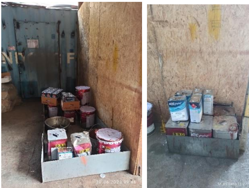
Figure 6. Chemicals/painting were stored with secondary protection at site of CC ZMEC (Status in May and June 2023)
