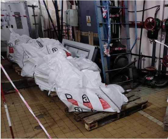
Figure 42. Removal of asbestos-containing debris and asbestos clearance work (Status in March, April 2023).
