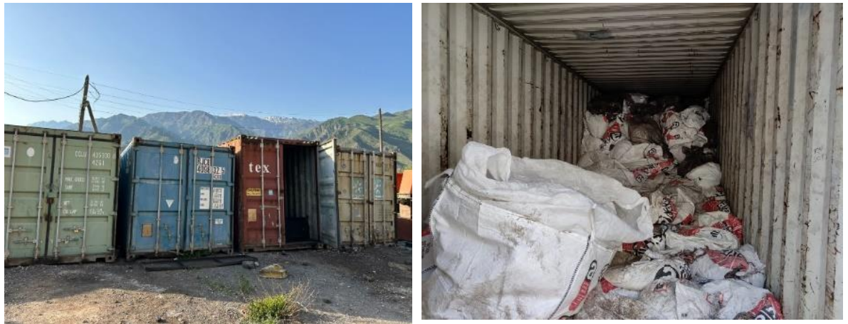
Figure 32. Collection of ACM waste bags and storage of asbestos waste at the designated storage area (Status in June 2023)
