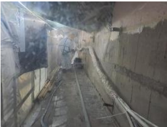
Figure 42. Removal of asbestos-containing debris and asbestos clearance work (Status in March, April 2023).
