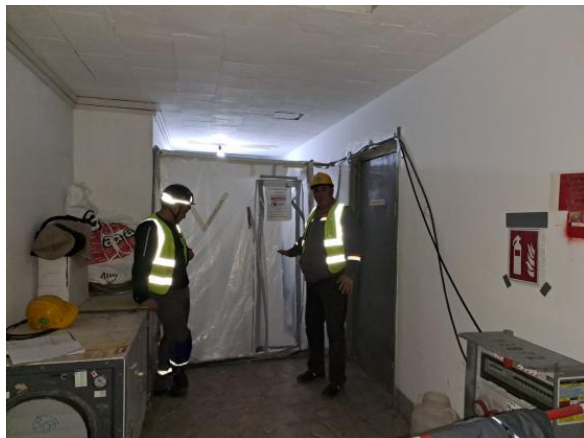
Figure 42. Removal of asbestos-containing debris and asbestos clearance work (Status in March, April 2023).
