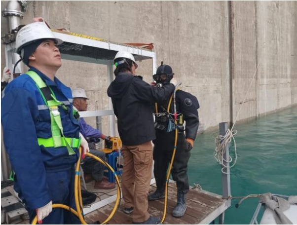
Figure 49. Diving work – installation of aeration pipes of a deep spillway under water (Status in April 2023)
