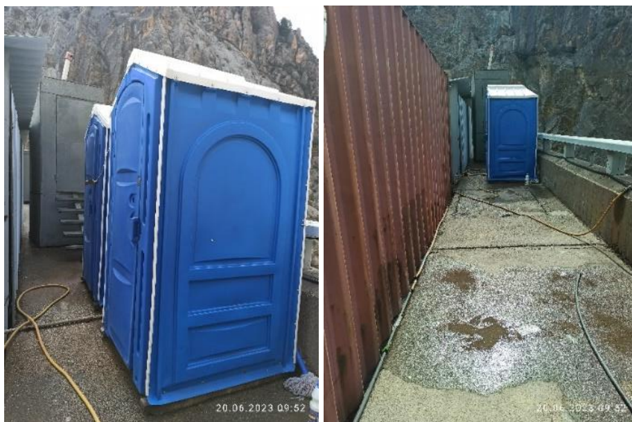
Figure 8. Portable toilets are available for workers working in the area of CC ZMEC (Status in June 2023)
