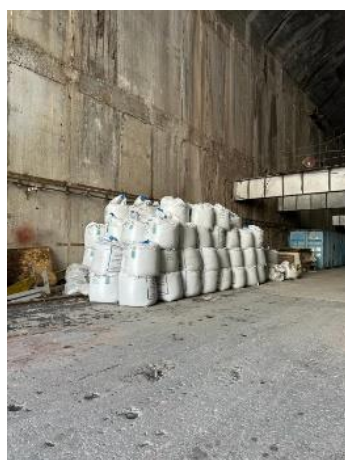
Figure 31. Temporary storage of abrasive waste at site of CC ZMEC and transportation for disposal (status in May-June 2023).
